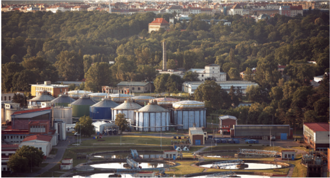
▲ A water treatment plant in Prague, Czech Republic. The Czech Republic's water supply and wastewater treatment services are highly privatised. ©Chalabala/Shutterstock
